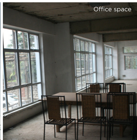
Finishing in progress
